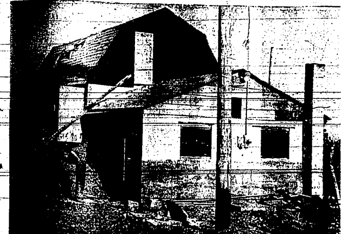
WAITING FOR COWS is Roy Rapp, Rapp and Dale Eden built the dairy barn to save money and time. The milking barn will handle 12 cows. Six are milked while six others are prepared for milking. The lower level houses the milk room and storage tanks. Milk is picked up every other day about noon. The door in the upper level leads to a 1,700-bushel feed storage room. Overhead storage permits easy feeding at milking time. (Times-News photo)
