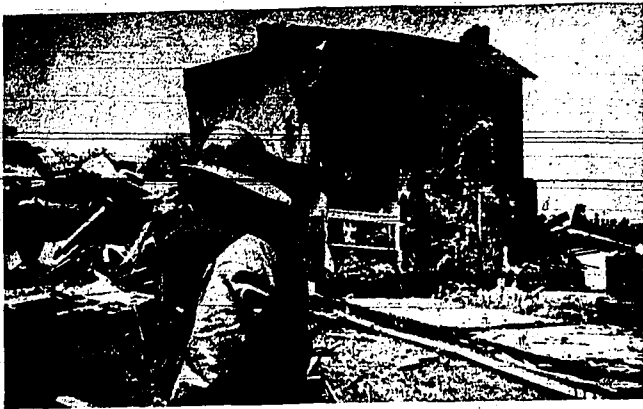
FIREMEN STAND in front of the ruins of a house that was struck by an F44 jet fighter plane near the Greater Pittsburgh airport. The plane struck the ground, bounced and smashed through the house. A portion of the fall can be seen to the right of the house while the cockpit is visible among the wreckage to the left of the house. (AP wirephoto)
