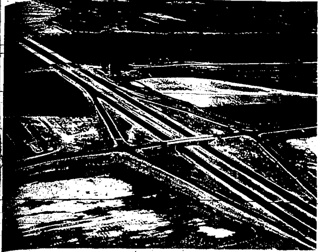
INTERCHANGE NEAR DECILO with Snake river bridge in background is detailed in this aerial photo of the district. It is typical of the great improvement being made in highways
