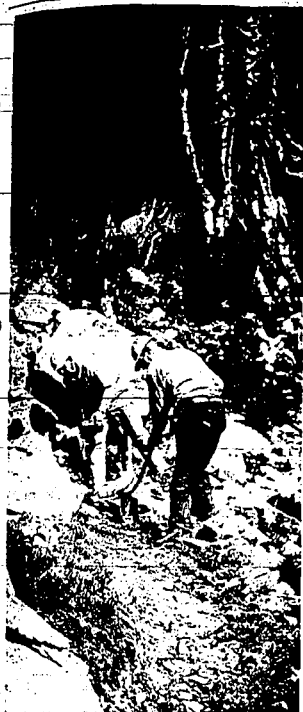
HARD AT WORK on a horse trail through the Sawtooth primitive area is a crew of forest service workers. After blasting some pick and shovel work to level the narrow pathway and make it suitable for travel by horseback, the forest service has a continuing trail improvement program in the area. This trail was completed last fall.
