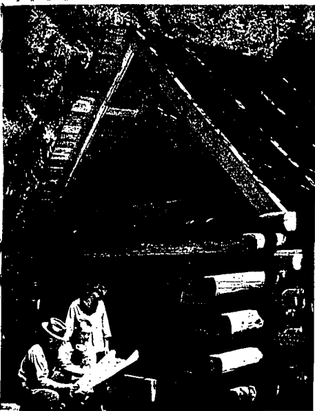
DISCUSSING THE FINAL phases of construction of one of the many summer homes in the Valley View summer home area of Sawtooth national forest is Jack Lavin, district ranger. The home under construction is the Munger home. Lavin and Munger check the blueprints to see if the building is being constructed as planned. Information concerning construction of summer homes is available from the forest service. (Forest service photo)
