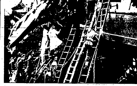
WRECKAGE OF TRAIN IN COLLISION NEAR MILLER, THURSDAY. A freight train hit a standing passenger train.
