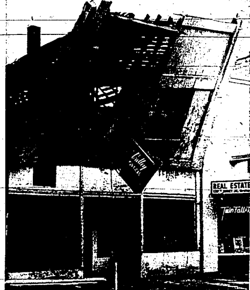
WALLS TUMBLE DOWN after the fire was extinguished in the 100 block of Main avenue east on Sunday morning. The walls were pulled down by crane to prevent them from falling and causing possible injury. The blaze started about 9:30 a. m. Sunday and was extinguished after a long fight. The building was completely destroyed. (Times-News photo)
