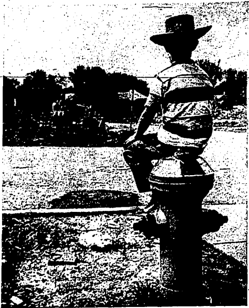
FIREPLUG FOREMAN Steve Johnson, 4, Des Moines, Ia., perches on handy seat to watch grading work on a freeway project near his home. (AP wirephoto)
