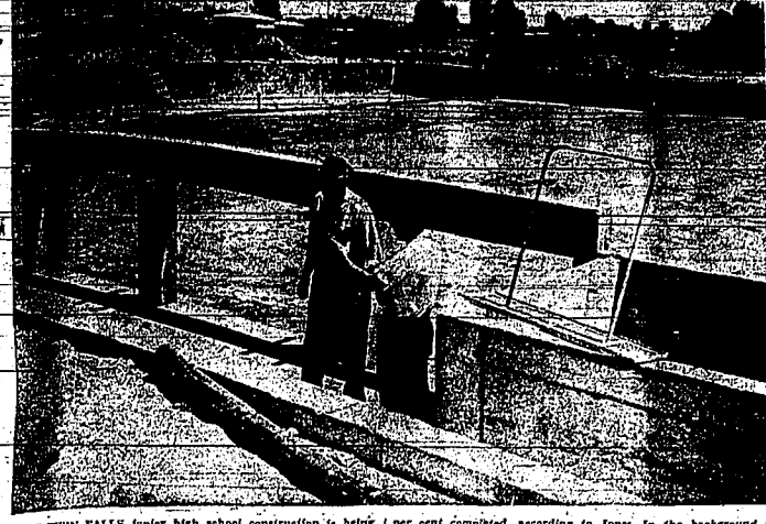
NEW TWIN FALLS Junior high school construction is being completed, according to Jones. In the background is the gymnasium area of the new school. The school is designed for about 300 students. Ragland says it will be ready for use in the fall of 1962. (Times-News photo)
