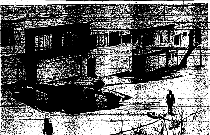
RAILROAD TUNNEL FIRE WHICH HAS BEEN BURNING UNDER ST. FRANCIS' PATRIOTIC HILL SINCE SATURDAY CAUSED THIS STREET TO CARE IN AND THREATENED THESE NEW HOMES WITH DESTRUCTION. The tunnel runs under them. Occupants of the homes have been evacuated along with those of at least 25 other homes built on top of the tunnel. (AP Wirephoto)
