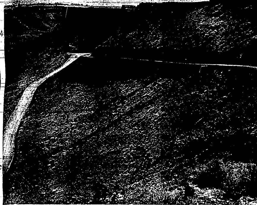
ENEMY OF CRYSTAL SPRINGS grade project is shown in this picture taken from the south rim of Snake river canyon. Replacing an old and dangerous grade, the new road makes easily accessible a vast recreation area now ready for use or under improvement. The grade was constructed by the Flieg highway district.
