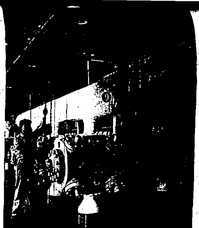
EL PASO NATURAL employs many Navajos in its operations. In this picture, Navajo employees are overhauling reciprocating compressor engines.
