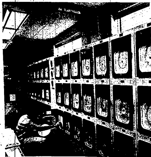
PIPELINE dispatchers maintain constant check on operations by means of pressure readings. These charts record gas pressures from different field locations.
