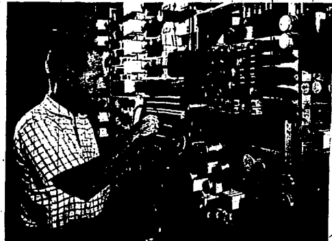
MICROWAVE units are used by El Paso Natural to maintain communications among offices and field plants or stations. This unit is being tested.
