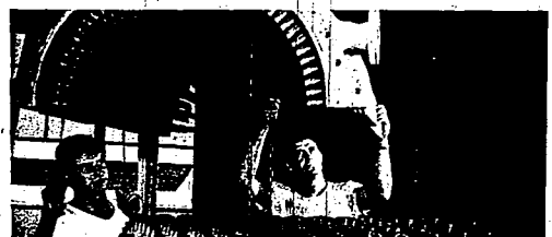
TURBINE STATIONS, in common with other El Paso facilities, are carefully overhauled to insure efficient operation.
