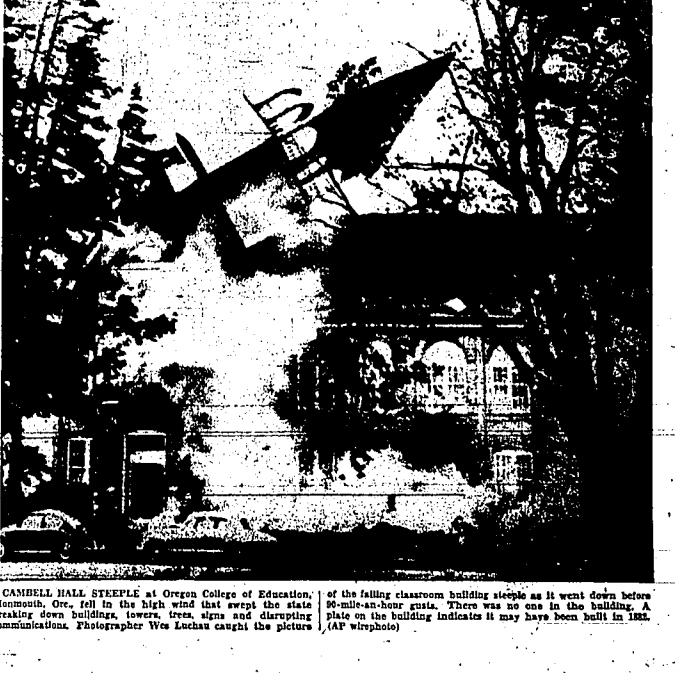
CANFIELD HALL EYEPLE at Oregon College of Education, Monmouth, Ore., fell in the high wind that swept the state...
