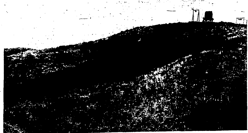
TONS OF EARTH are moved by a barely seen bulldozer as a ski run at Soldier Mountain is prepared for winter use. The popular area, located some 10 miles above Fairfield on the mountain's east side, was started 12 years ago.
