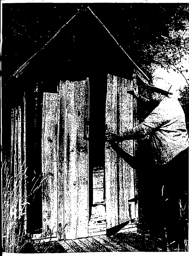
MORE ACTIVE HALLOWEENS, now long past, were in the mind of J. A. Cederquist, Twin Falls business man, when this picture was snapped. This would put the time of the original picture back about 1907 for Cederquist, who recalls the practice was a frequent, but not appreciated by the owners' pastime.
