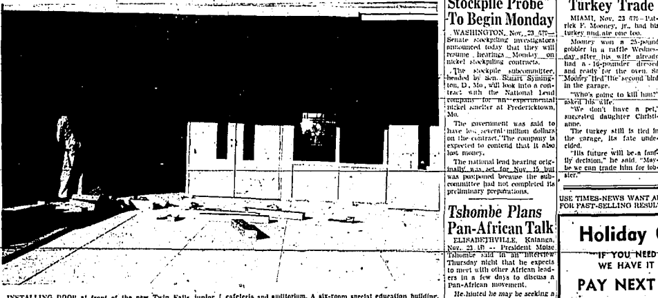
INSTALLING DOOR at front of the new Twin Falls junior high school building is D. M. Westrich, employee of the J. A. Clawson Construction company, Twin Falls. The building includes a gymnasium, library, 23 classrooms and a combination cafeteria and auditorium. A six-room special education building, where handicapped children will be taught, also will be built next to the junior high school building which will be ready next fall. (Times-News photo)
