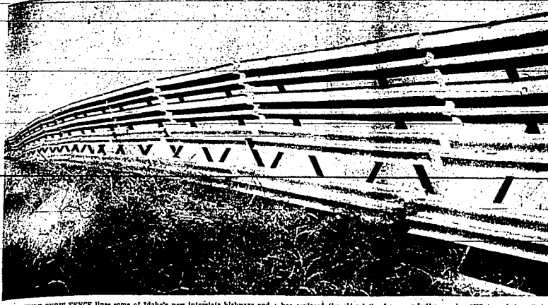
NEW TYPE SNOW FENCE lines some of Idaho's new interstate highways and has replaced the older lattice fence and the wooden "X" type before that. It is made of heavy-duty steel pipe and is designed to last for many years, without any continuing cost for upkeep. (Times-News photo)
