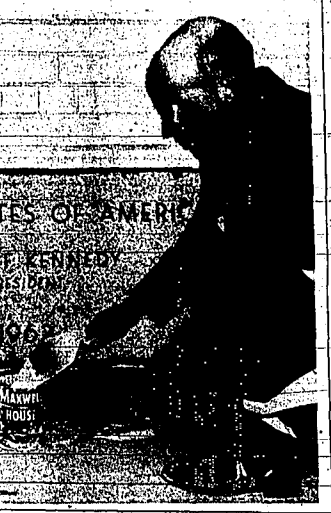
Research center. They applied the final mortar around the cornerstone during the cornerstone laying ceremonies Saturday afternoon. About 80 persons braved the cold winds to attend the event. (Times-News photo)
