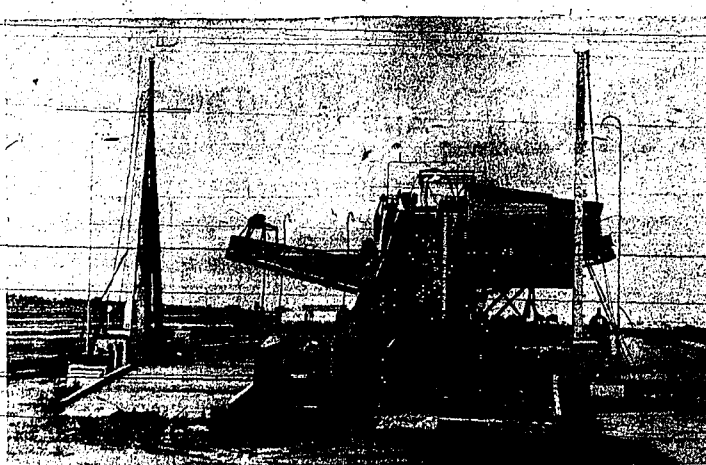
SPEEDIER operations are expected at Amalgamated Sugar company beet dump at Curry. A new dump and piler has been installed. A key feature is the method by which the dirt is returned to the farmer's truck. The dirt conveyor works right off the left and the farmer drives off the platform directly under the conveyor to receive his dirt. (Times-News photo)
