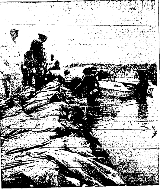
VOLUNTEERS UNLOAD SAND BAGS brought by boat to reinforce a weak spot in the levee at Port Aransas, Tex. Many of the community's homes were flooded by two levee breaks which have been repaired by the volunteer sandbagging. (AP wirephoto)
