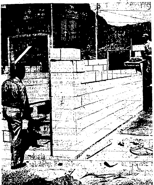
RESTROOMS AT SHOSHONE falls park are being constructed by Twin Falls parks and recreation department crews. Working on the 20- by 10-foot cinder block building are Paul Monigery, left, and Clyde Biggers, right, while Howard Johnson, center, departmental superintendent, looks on. The restroom is being built along the main road leading to the parking lot, near the turn-off to other parts of the park. (Times-News photo)
