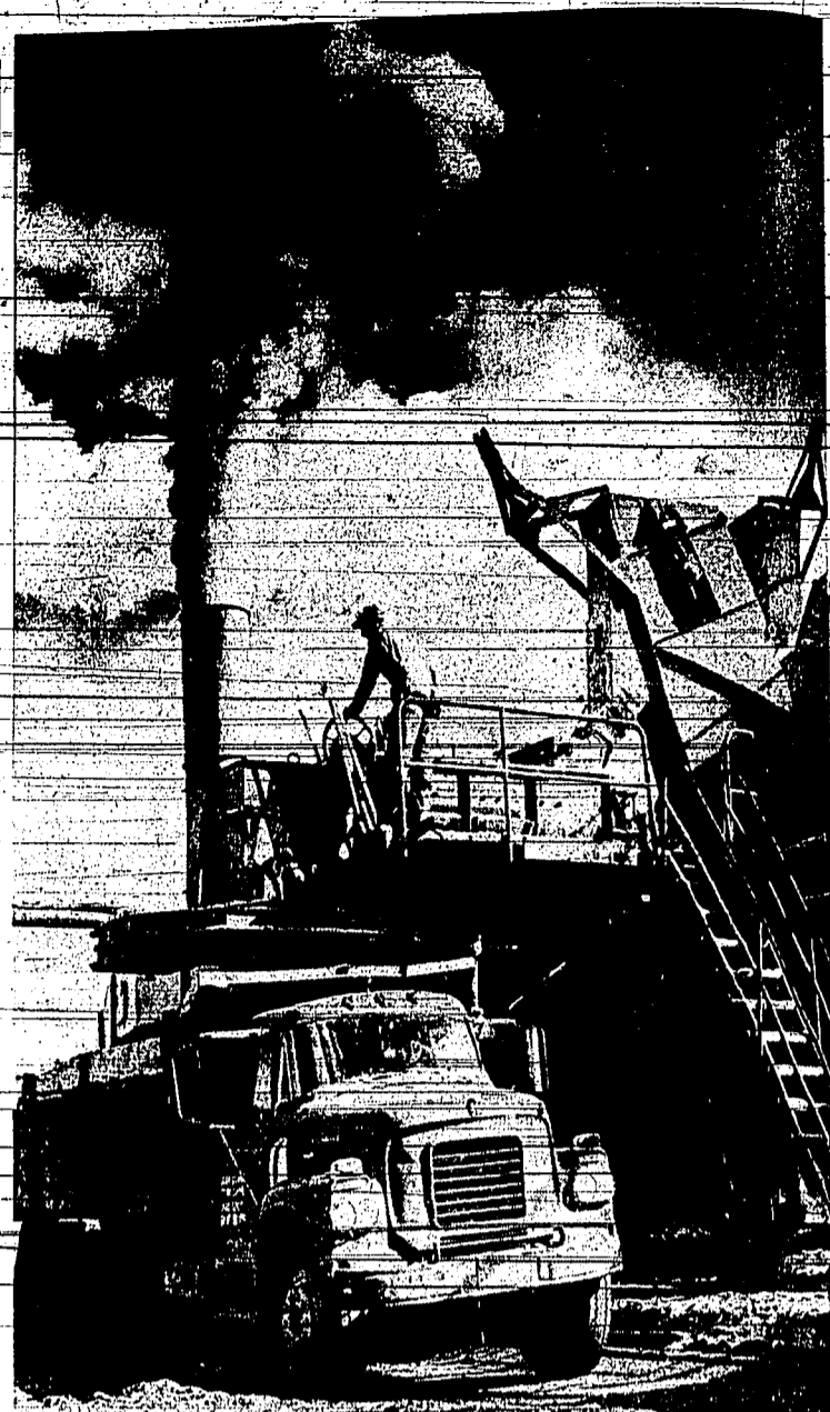
SMOKE LEAPS SKYWARD —as "puffing Betsy" goes about the work of being a part of the mixing equipment utilized in construction of highway 30 east of Twin Falls. A truck waits under a belt mover while mix is dumped for the trip in the road section being completed. Modern equipment such as this assures construction jobs speedy results. (Times-News photo)
