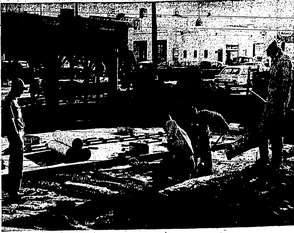
CONSTRUCTION ON THE new Idaho Power company office, to be located at 133 Third street north, is getting under full swing. (Times-News photo)
