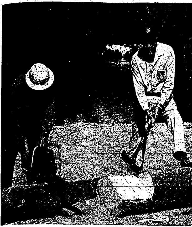
FRANK LANHAM, Coeur d'Alene, maintenance man (with axe) and James Archer, temporary driver, work on log auto barrier separating parking area from picnic grounds at Rose lake in Kootenai county. Both are with the Idaho fish and game department. This development work was an accelerated public works project and the Rose lake access area will be maintained by Kootenai county workers.
