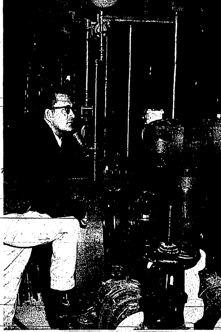
INSPECTING COMPRESSORS is W. W. Paulson, Burley businessman. Paulson installed two 75-horsepower compressors to freeze the ice on a new rink he constructed on the north side of Burley. The ice will be frozen artificially by piping ammonia gas through brine pipes buried in a concrete slab. The rink measures 85 by 185 feet and is the largest outdoor rink in Magic Valley. The machinery to freeze the ice is housed in a separate building behind the rink. (Times-News photo)
