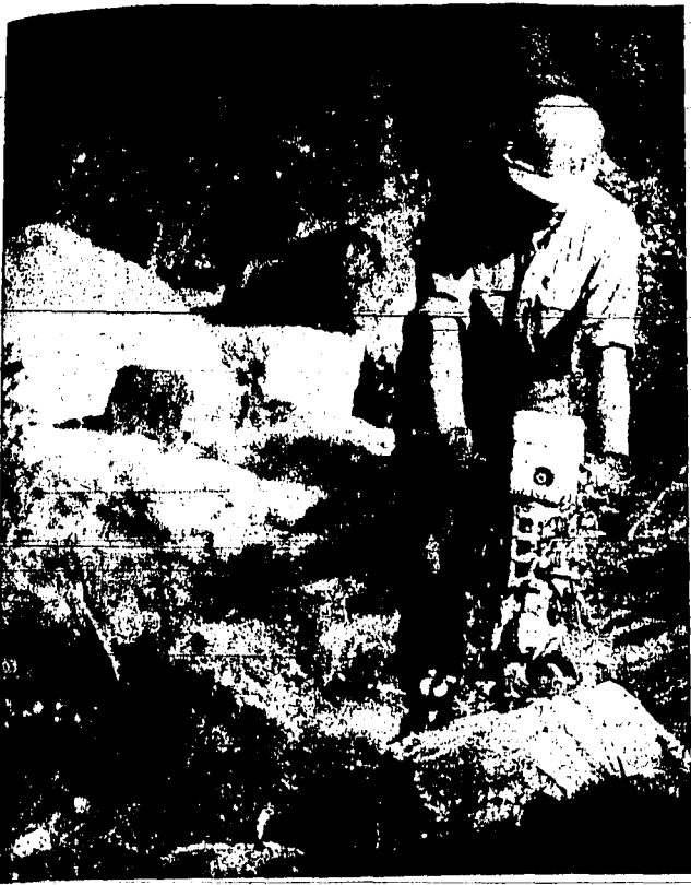
WORKER IN CHALLIS national forest is shown drilling into rock prior to blasting operations on Loon creek trail. Trail making and cleaning is becoming a major job in all forests. (Forest service photo).
