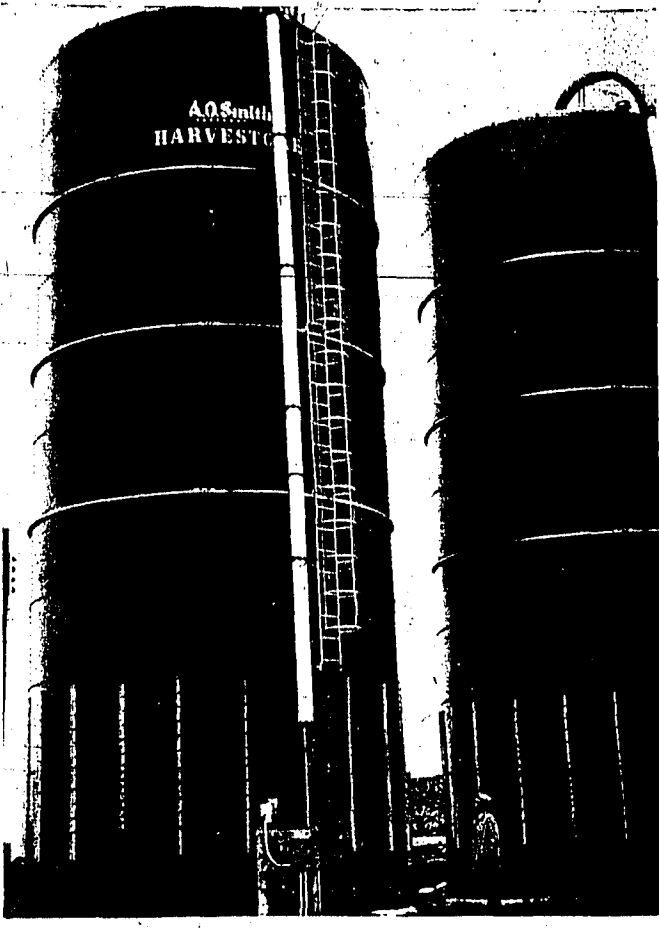
NEW GLASS-LINED silo is examined by M. O. McVey, who recently acquired a franchise to market the new product in the Intermountain area. The new silos, located about six miles east of Hazelton and a mile and one-half north, are near the railroad siding of Schodde. The farm is owned by Dr. Ben K. Humphreys, Rupert. (Times-News photo)
