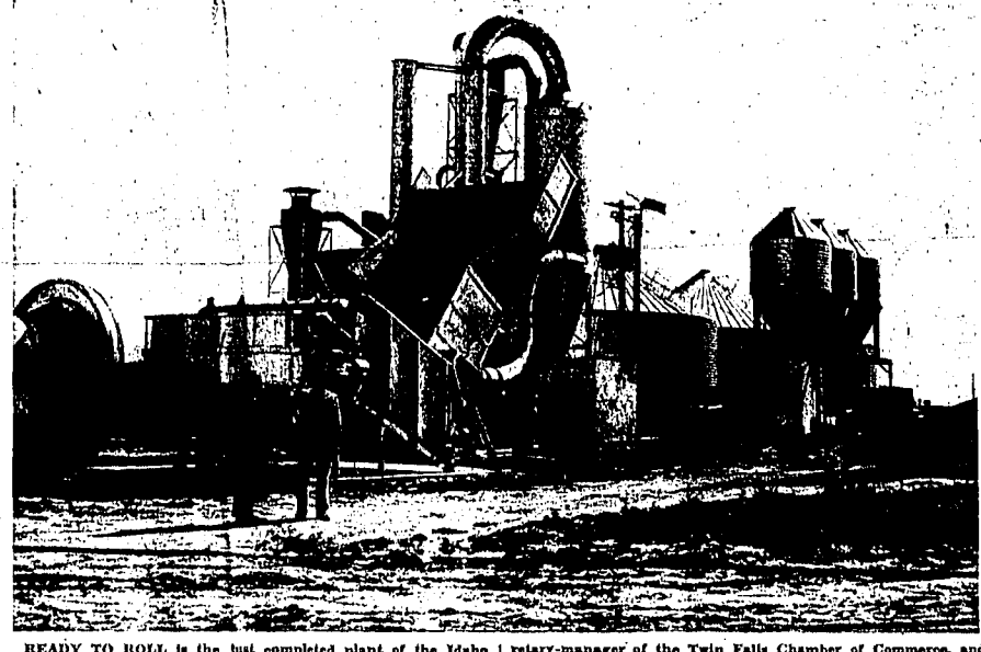
READY TO ROLL is the just completed plant of the Idaho Alfalfa Products company, only setup of its kind within a 400-mile radius of Twin Falls. Preliminary operation tests were to be completed this week, with actual operation on a production scale getting under way Monday morning. William Grange, left, secretary-manager of the Twin Falls Chamber of Commerce, and Beryl Lemmon, plant owner, discuss the setup during testing. Pellets from green and baled alfalfa will be manufactured at the facility, located east of the city near the sugar company plant. (Times-News photo)
