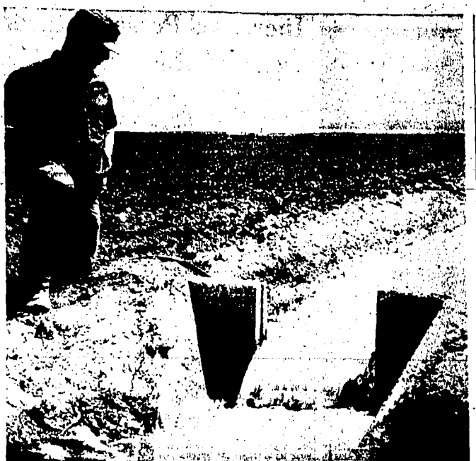
SUCCESSFUL WATER management is demonstrated by Douglas Schroeder, Salmon tract farmer. New ditches were laid on the Schroeder farm utilizing a check gate and siphon tubes. The ditch has a minimum fall between check gates. Flow is controlled by splash boards. The irrigation flow is set up on quarter mile runs and Schroeder can change the water in the time it takes him to walk the field. The system eliminates hours of irrigation work and wasted water. (Times-News photo)
