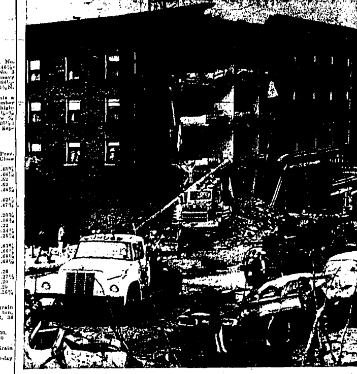
HUGE EARTH-MOVING rig crushed two cars, then smashed into a four-story hotel in central Seattle. The rig, described as a 'turnip', was partly buried in bricks that showed from the Panama Hotel.
