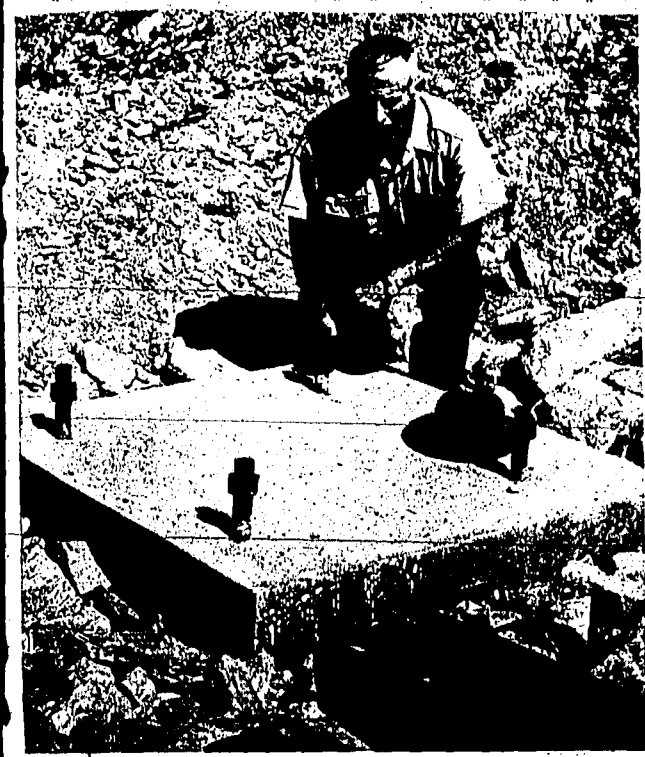
CEMENT BASE for one of many towers for the new double chair lift at Pomerelle is built for rugged use. District Ranger Merlin Block, shown inspecting one of them, said that the cement is poured to a depth of about seven feet and the base itself is four by five feet at the top. The towers of the ski lift are anchored to this base. The main base, at the bottom of the hill, is many times larger than these which extend to the top. (Times-News photo)
