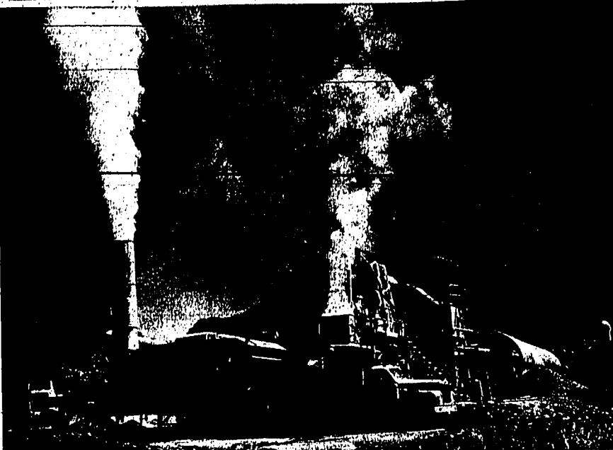
ASLETT CONSTRUCTION COMPANY, Twin Falls, is operating this busy asphalt mixing plant at Big Bar on the Snake river to provide surfacing material for Idaho Power company's new access highway to the Hells Canyon dam site. Gravel for Aslett's extensive paving work in North America's deepest gorge is being produced at two other rock-crushing plants, one several miles from the asphalt plant and one at Oxbow. The Twin Falls
