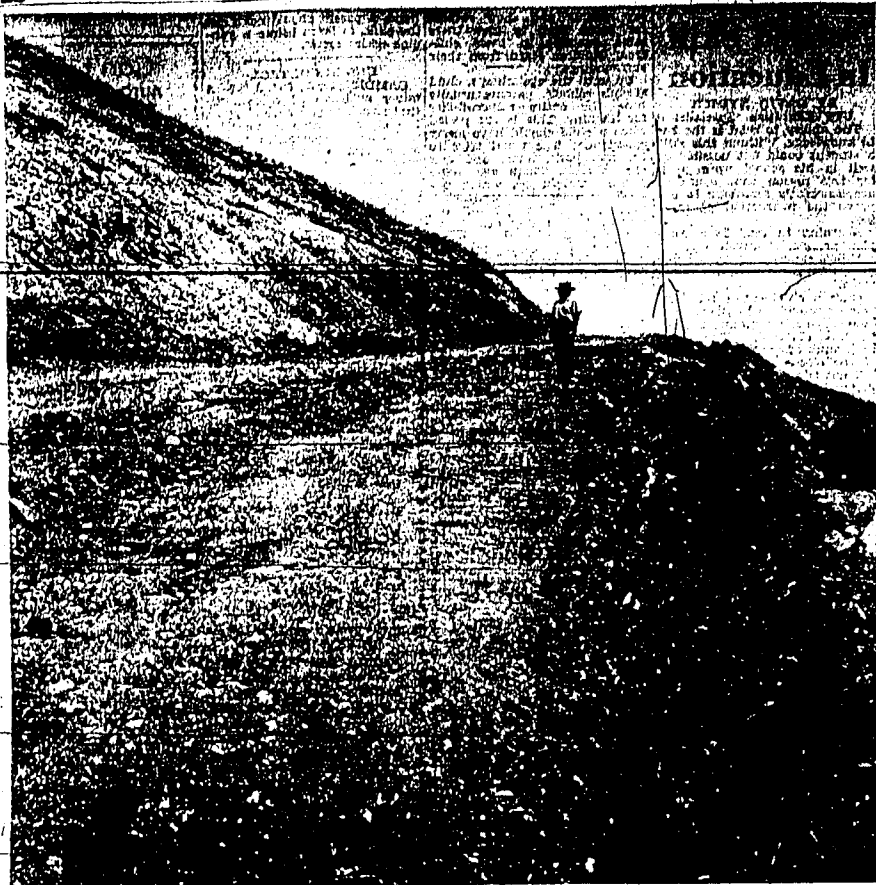
NEW ROAD FOR the Pomerelle ski and recreation area south-east of Burley will make the old one look like a pioneer trail. Being rushed to completion so it can be used this winter, the road is set for oil surfacing next year. It eliminates many curves of the old road and permits snow to be pushed over the edge. It will permit operation of the ski facilities several weeks longer next year because it will permit easy access. Merlin Stock, Burley district ranger, is shown on the road. (Times-News photo)
