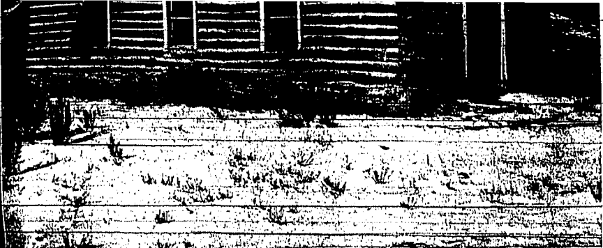
NO LONGER echoing to the shouts of students, the log Moulton school stands deserted and practically forgotten, a victim of progress. Only the shell of the structure remains, the desks and interior fittings having long since been carted away by passersby.
