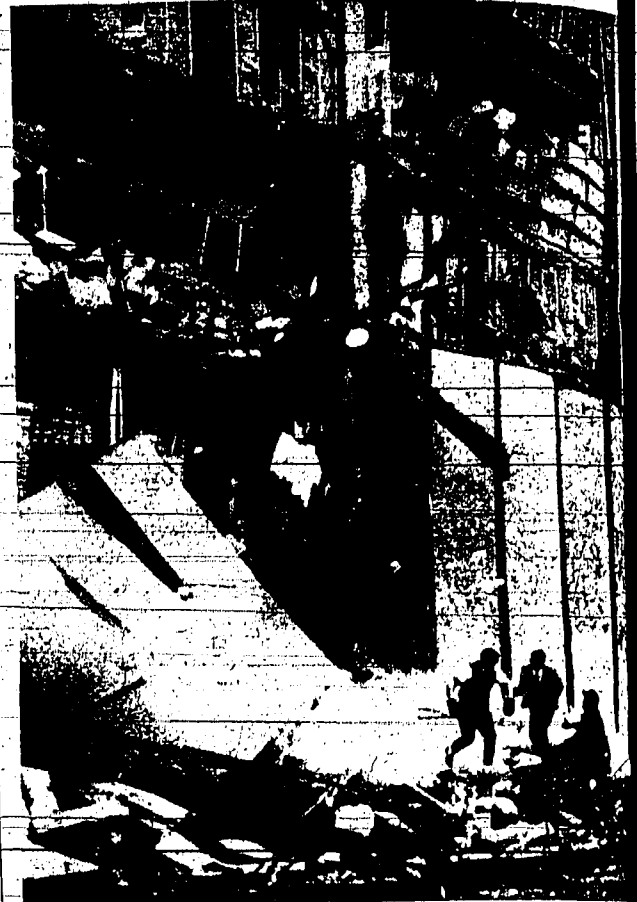
WALLS OF A FIVE-STORY building crash to the street after they were shaken by force of an earthquake that struck Anchorage, Alaska, in March. This photo was made by Iyohetnik of the Anchorage Times. (AP wirephoto)
