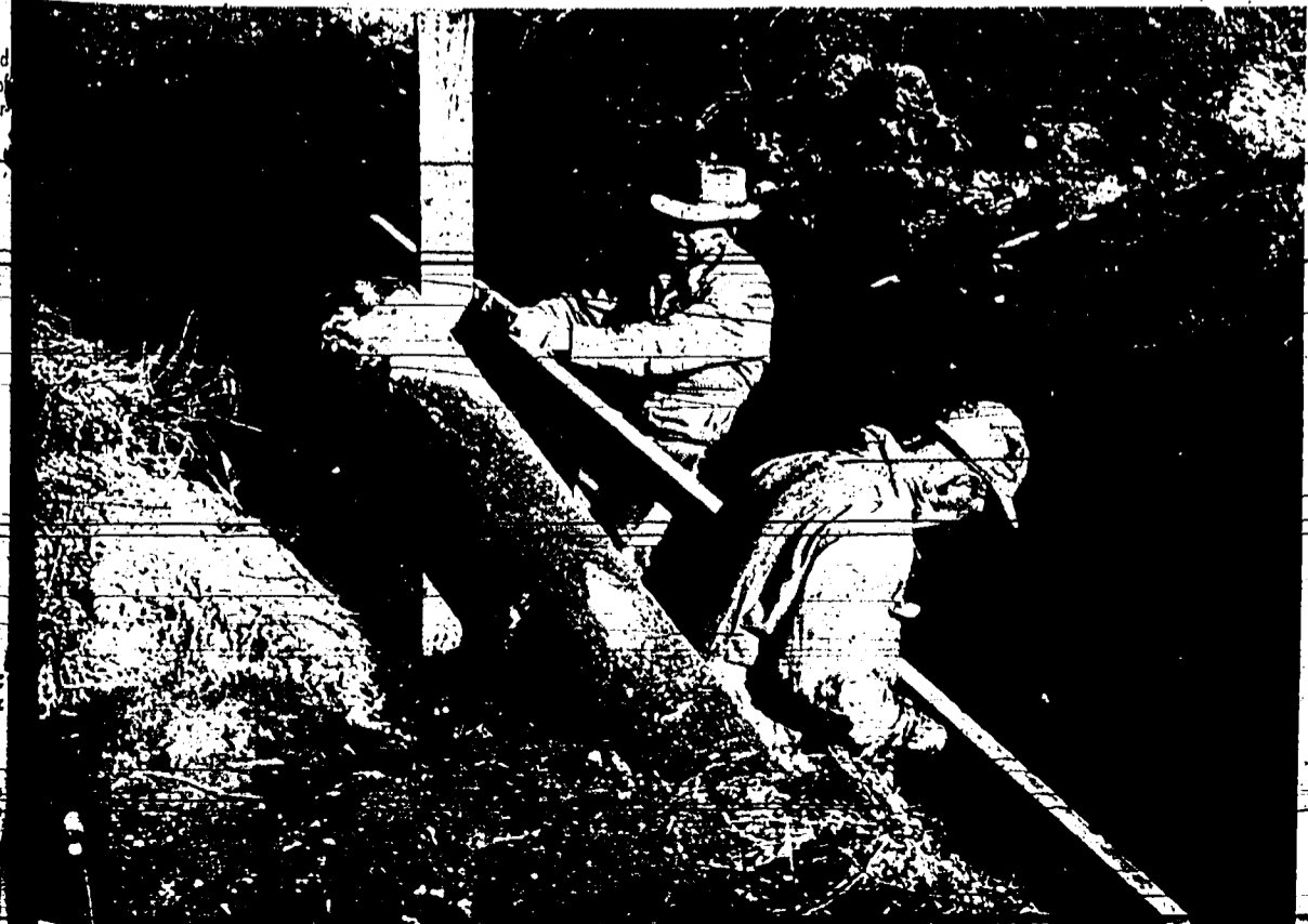
DEEP IN MUD and water are Frank Thietten, near end of pipe, and Vernon Smith, as they install a 10-inch pipeline which will carry water back to the head of the fish runs at Rock creek Hatchery. Thietten was chairman of the project and Smith is chairman of the board
