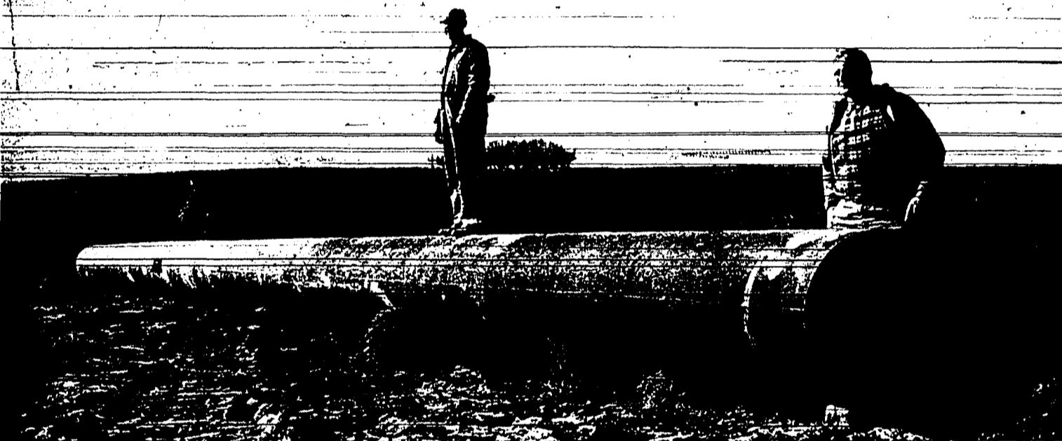
NINETY-FIVE FOOT LENGTH of pipe, after joining of the various sections, is ready for lowering into Salmon Falls creek canyon. Two men holding responsible positions in the Magic Water company and long involved in the development of the new irrigated area, stand by the pipe. In the foreground is Maurice H. Eckert, vice president of the company, while Asa T. White, manager, is in the background. There are six farms in the new area.
