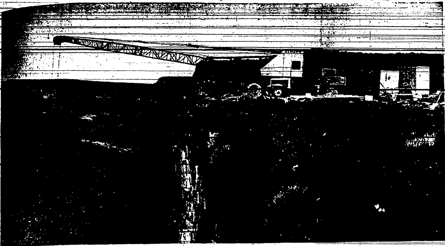
MOST MATERIALS needed in construction of a new irrigation pipeline for the Magic Water company must be let down into the Salmon Falls creek canyon by means of this large crane. Probably the heaviest piece of material to be lowered will be a piece of 30-inch steel pipe, 95 feet long and tipping the scales at about 10,000 pounds. The vertical drop involved is more than 100 feet, while the pipe from water source to canyon rim will be 710 feet. (Times-News photo)
