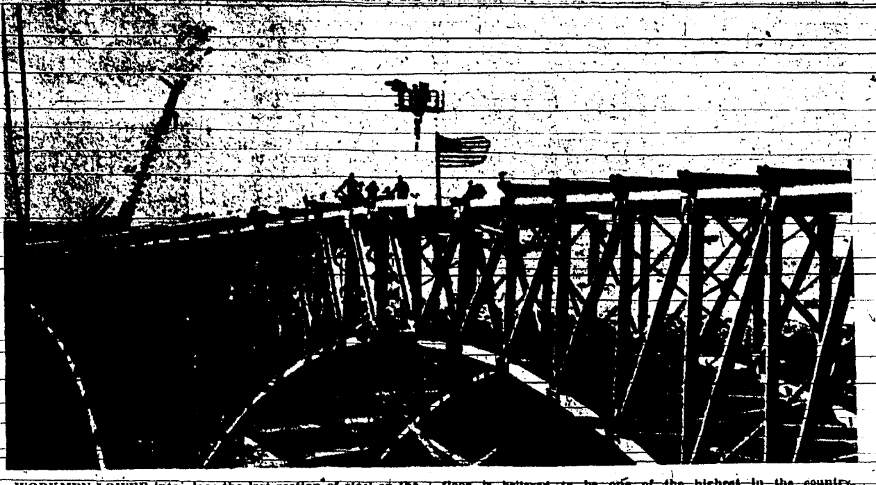
WORKMEN LOWER into place the last section of steel on the Rio Grande gorge bridge, which, at 650 feet above the canyon floor is believed to be one of the highest in the country. A ceremony marks the placing of the last piece. (AP wirephoto)
