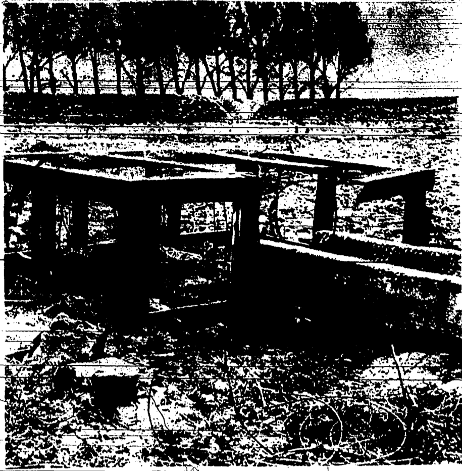
THIS EARTH RESERVOIR is a historical landmark in the water system of Twin Falls. Constructed in 1918, it stored the water for the city until 1939. Shown here is the drainage point, where the water was carried to the filter plant, just west of the reservoir. (Times-News photo)
