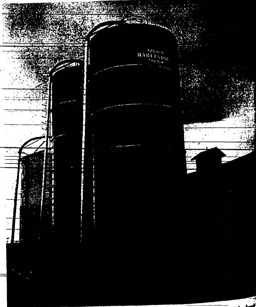
These two 20-by-60 foot "Oxygen-Free" Harvestore structures are the heart of Mr. Garrard's automated feeding program. Harvestores are so constructed to completely eliminate feed spoilage and loss.
