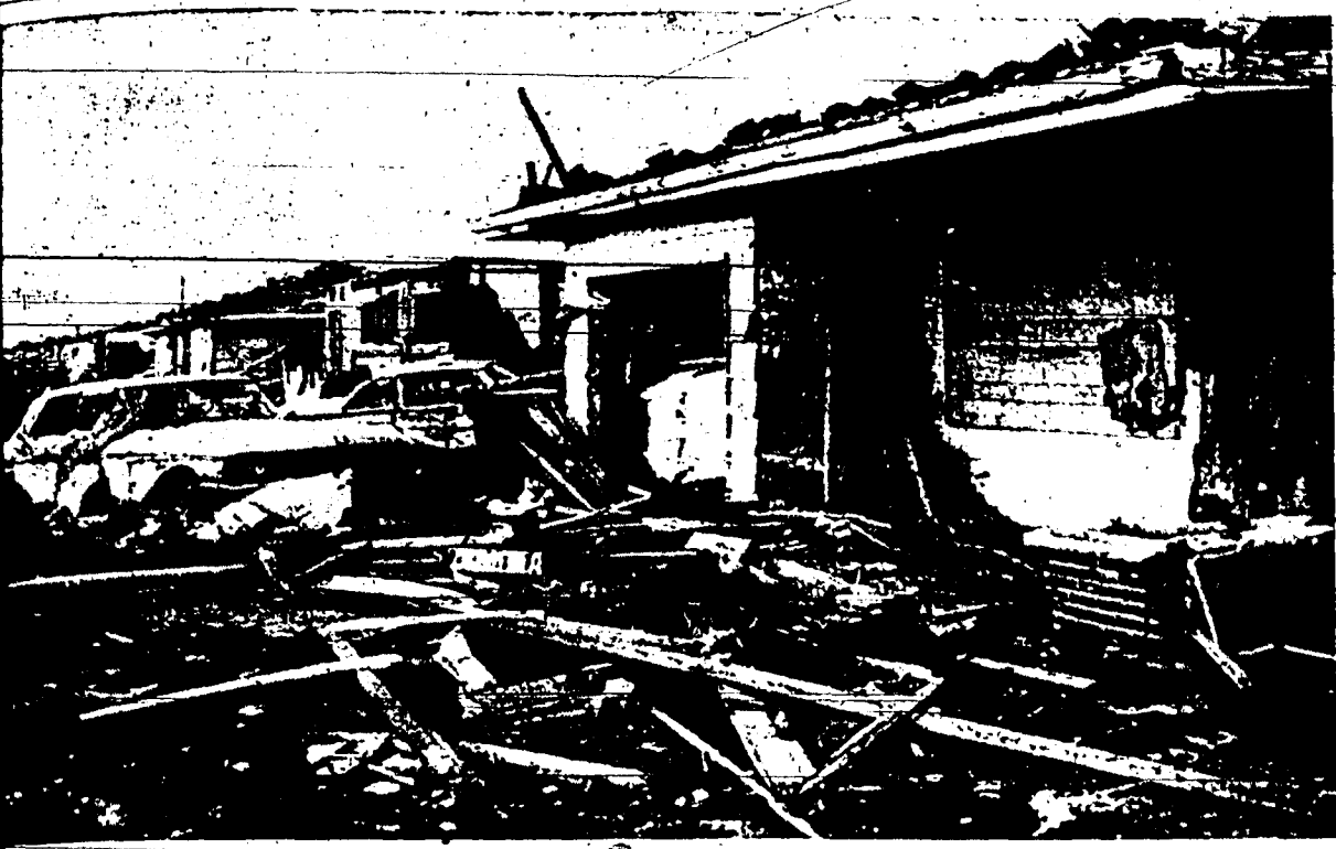
UNROOFED BUILDINGS and scattered lumber are everywhere visible in this subdivision of Colby Estates, Crystal Lake, Idaho, which was hit by a tornado late Sunday. Tornadoes smashed
