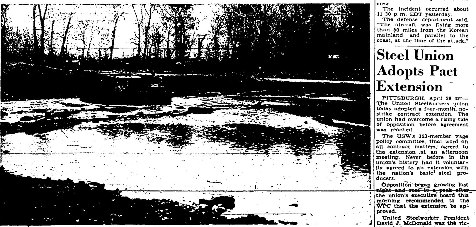
WORKMAN FOR THE Mike Erie Construction company works against time to push back 5,000 cubic yards of river gravel onto a bank to keep waters of the Big Wood river, seen in background, from flooding ranches in the Broadford area near Halley. The Wood River Valley Irrigation district is widening the main channel of the river to take pressure off the east bank of the river which, if water overflows there, would flood the Bellevue city park. This silting pond of gravel has been formed to assist with flood control of the river. The dam is several hundred yards from the canal company's diversion dam. Some 200 feet of retaining wall has been built along the east bank of the river above the headgates of the district canal. (Times-News photo)
