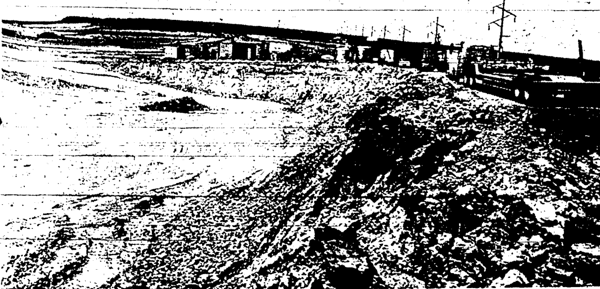
THOUSANDS OF YARDS of soil is being removed from this site for use as fill in construction of the interstate highway in the area of Jerome and Hazelton. Repair sheds for heavy trucks in the work also are maintained at this point. Traffic into and out of this pit is so intense that a special stop and go light has been installed at the entrance, blocking private traffic as heavy trucks speed to the dump location. A workman operates the light. (Times-News photo)
