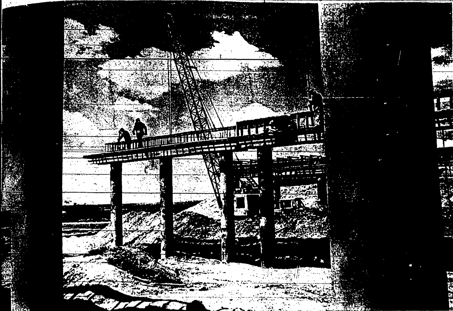
GREAT CEMENT support posts of interchange on highway 80N north of the Hansen bridge makes a dramatic photograph of construction now being worked in that area. Workmen can be seen on top of one of the support beams while a great crane, used in the lifting work, is noted in the background. Motorists will speed through this area at 70 miles an hour, with unobstructed vision and few curves, when the highway is completed. (Times-News photo)
