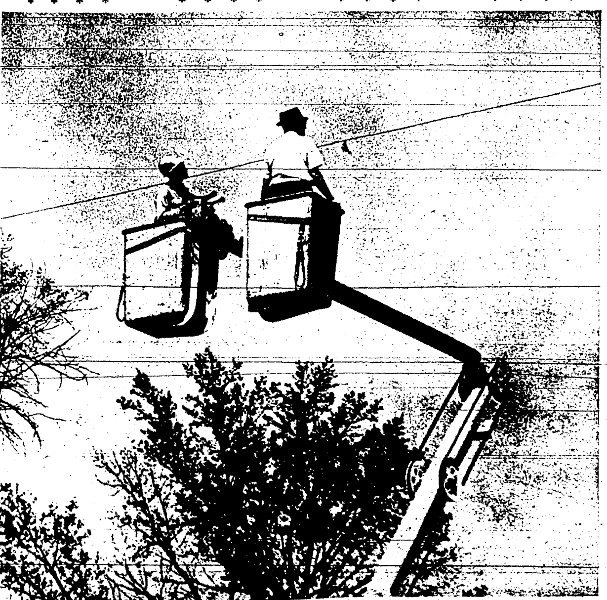
POWER COMPANY official, Earl Haroldsen, right, is hoisted aloft to get a close look at the bird on the wire. The Idaho Power Co. "cherry picker" enables the close inspection. The
