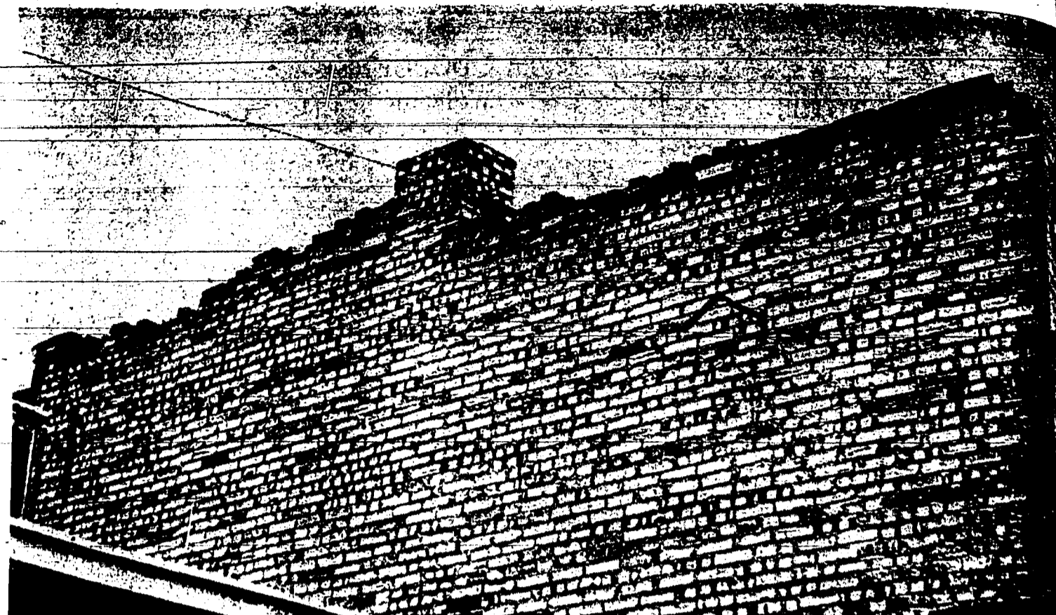
TOP OF WALL on this downtown building is unstable. Bricks are loose and a building is given as being between 30 and 50 years, depending on type of construction. (Times-News photo)
