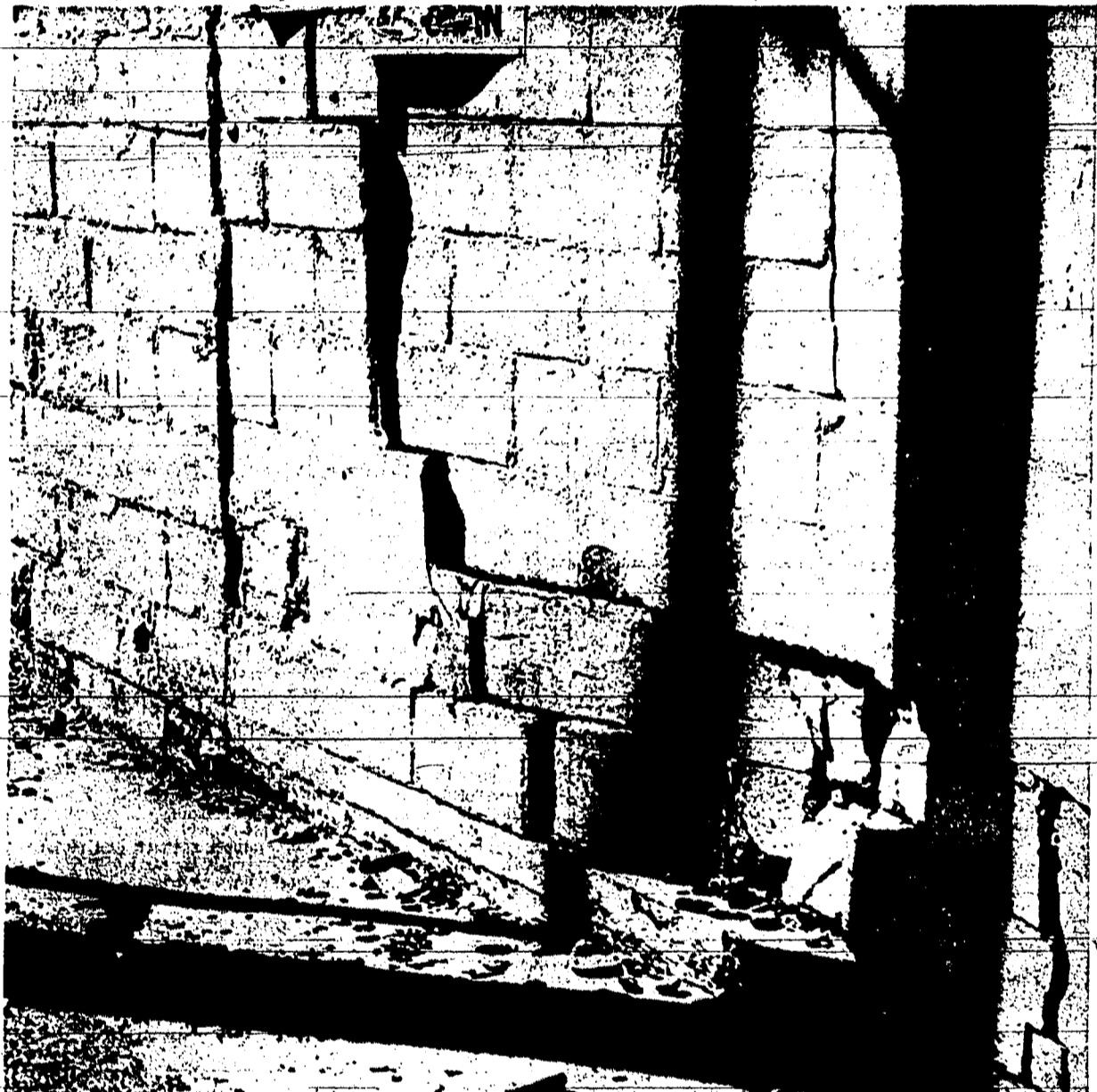
AUTOMOBILE or truck came out the winner in a bout with the wall on the back of a downtown structure, as this picture shows. Someone parked just a little too close, with the result a near cavern resulted. (Times-News photo)
