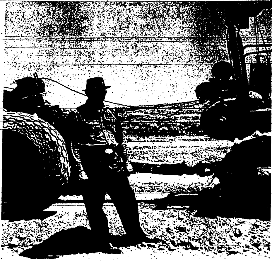
WORK BEGAN Tuesday on a new 12-boy unit at the Idaho Youth Ranch at Rupert. Rev. James Crowe, superintendent, supervised removal of ground. This is the second new unit to be constructed at the ranch, but will make the third home unit as an older house has been converted into a living unit. Applications are being taken for house parents for one of the units. Rev. Mr. and Mrs. Crowe will move into Rupert once the new house parents have been chosen. (Times-News photo)
