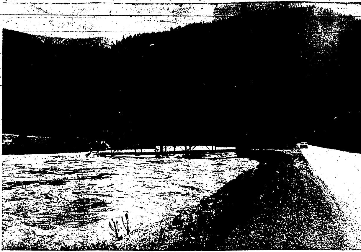
ONLY HALF OF a bridge crossing the Salmon River from U. S. Highway 93 near North Fork remains standing. Section was carried downstream as river hit record high Sunday night.
