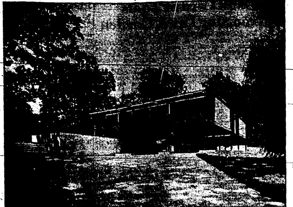
NO INSIDE COLUMNS in this home. The variety and versatility of modern steels are solving home design problems, so this house could be erected on a narrow, deep lot. The steel frame is composed of star columns consisting of four steel angles spaced two inches apart. Beams are built-up tubes of steel plates with continuous bar separators. Tubes are placed between angle columns, forming a frame, which permits complete freedom of planning within the house, since there are no inside columns.
