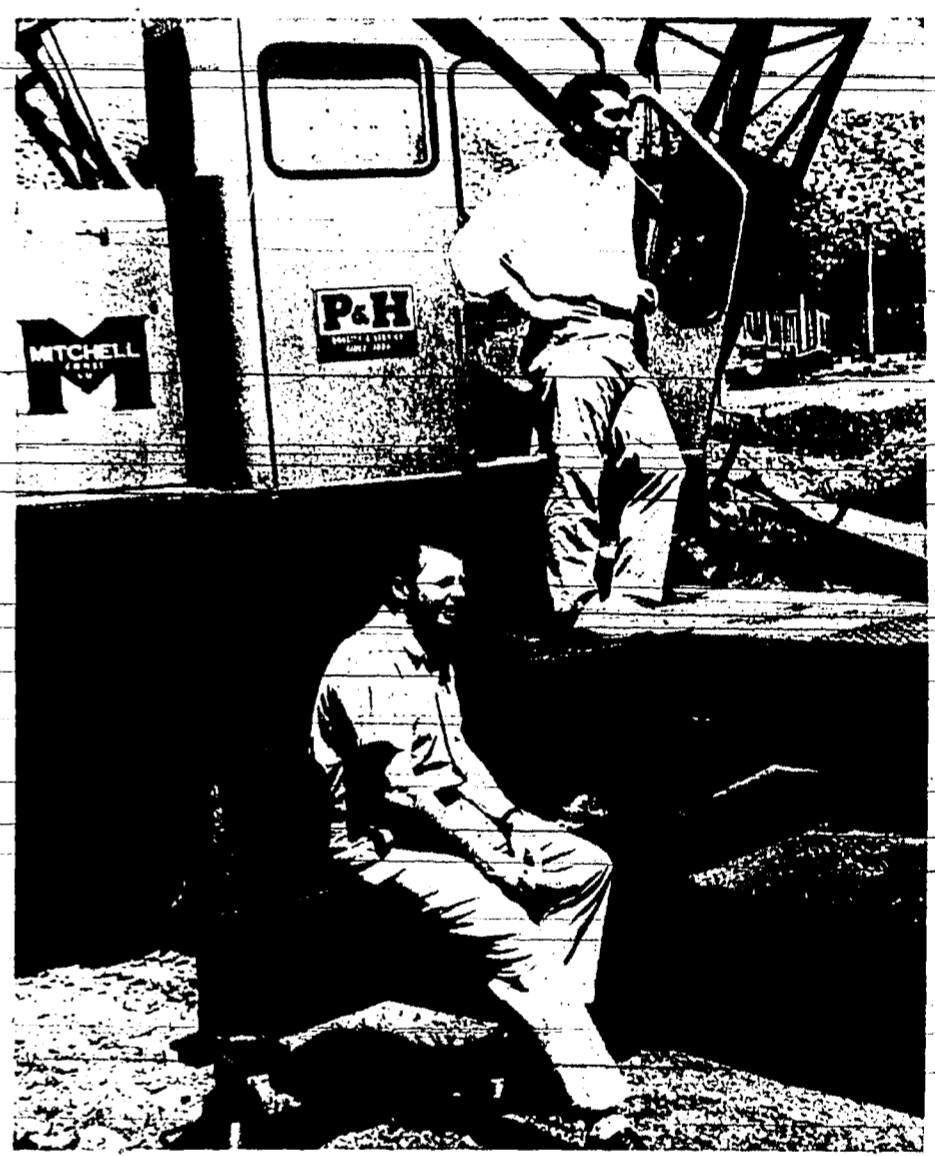
GIANE CRANE is background for Fred Beck, director of marketing and publicity and David Jay Flood, architect-in-residence, at the site of the Sun Valley expansion project. The crane is part of the heavy equipment used by the Mitchell Construction Co., Pocatello, in the crash program to get the facility built by Dec. 15. (Times-News photo)
