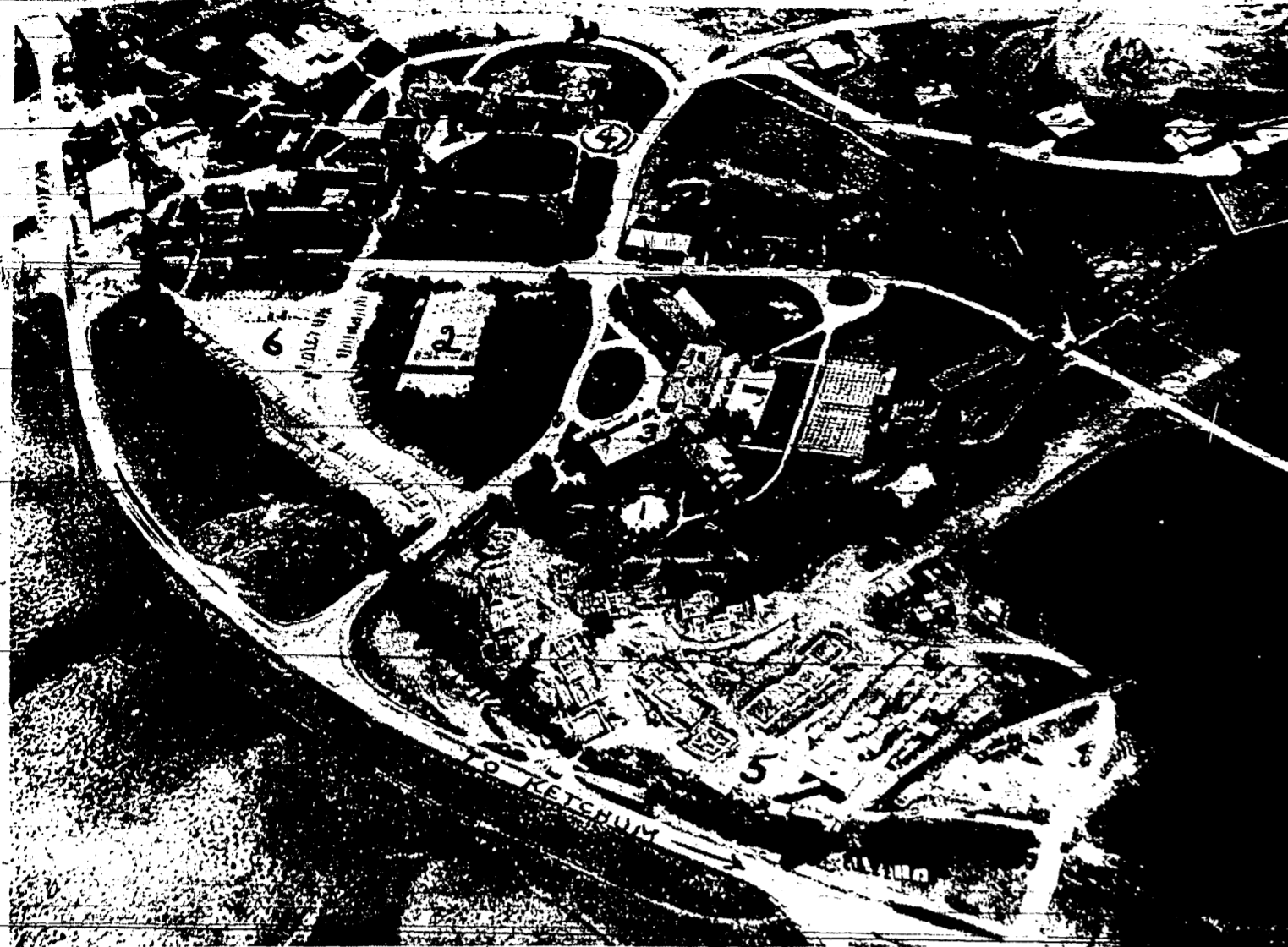
AERIAL VIEW of Sun Valley, taken last week, gives graphic picture of entire area including site of new Lodge Apartments, 50 in number, now being constructed. In the picture, area 5 is the apartment site; 6 is one of several parking areas; 2 is the tennis courts; 1 is the Sun Valley Lodge swimming pool; 4 the Challenger Inn swimming pool and 3 is the lodge. The main road on the
