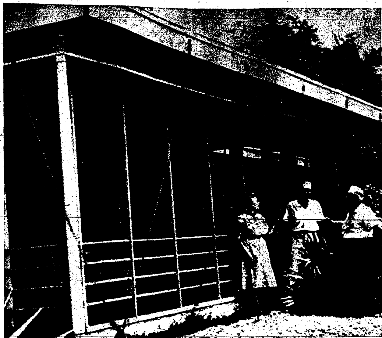
READY FOR HURRICANE is this house in Panacea, Fla. Fred Yoars, center, and his wife stand under the overhang of their chained roof as they explain how their residence rode out a tornado that unroofed a half-dozen other houses and smashed a warehouse in their vicinity last year. The flat roof is secured all around with lengths of quarter-inch chains anchored to steel bolts imbedded in the concrete foundation. The Yoars feel certain the chains and other reinforcing steel straps inside their house can withstand winds of hurricane force. At right is Capt. W. S. Schley, Civil Defense aide. (AP wirephoto)
