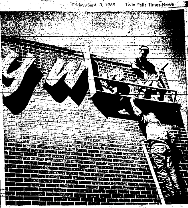
SHOWN WORKING ON YWCA sign are Richard Connor and Mrs. Don Lambert. Mrs. Lambert made this sign, and also a YWCA sign to the left of it, not shown in the picture. Both signs are made from styrofoam plastic, painted and glued to the front of the building with a strong cement. The signs took three days to erect and provide the finishing touches to the building. (Times-News photo)
