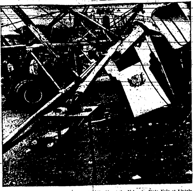
HUGE STAKES BRACING a cable car Sky Lift ride at the Nebraska State Fair at Lincoln, were uprooted when two of the ride towers fell over Sunday, dropping passenger gondolas more than 30 feet into the crowd below. At least two persons were killed and 50 injured. Shown at right is the Sky Lift ticket booth. (AP wirephoto)
