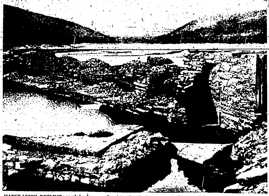
WATER LEVEL DECLINE revealed a former railroad trestle in Whittingham Lake at Wilmington, Vt. During high water periods the railroad trestle is completely under water. In days gone by, it was used by the Hoosac Tunnel and Wilmington Railroad. In the foreground is a section of Mountain Mills Paper and Pulp Co., which began business in the early 1800s. The lake was formed in 1921 by New England Power Co. to generate power for New England. (AP wirephoto)
