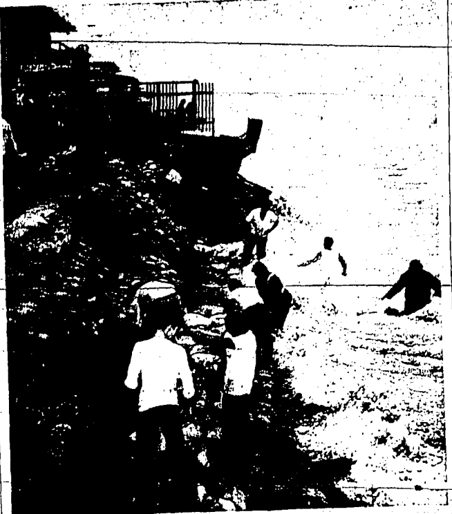
WORKMEN PILE SANDBAGS to reinforce the seawall at Capitrano Beach, Calif., Monday as high tides continued to threaten homes on the Southern California ocean front. Prisoners from four Forestry Conservation camps were working beside forest rangers, county crewmen and volunteers in their fight against the sea. (AP wirephoto)
