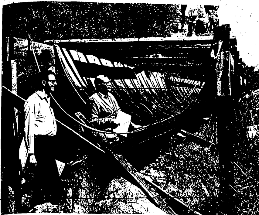
OLD FLUME, which for years carried water to irrigated lands below, is inspected by Forrest Closser, left, area conservationist from Pocatello and Clarence Hedrick, unit conservationist, Soil Conservation District, Twin Falls. An underground concrete pipe now replaces the flume from which much of the irrigation water escaped before it reached the farmlands. It is planned to remove the flume from the canyon. (Times-News photo)
