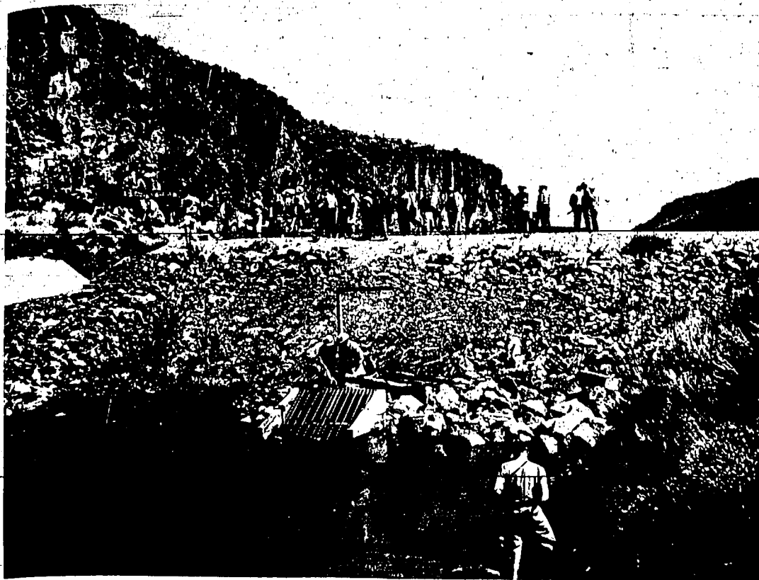
INSPECTION TOUR members visiting the Cedar Creek watershed project gather atop the new diversion dam which results in irrigation water being directed into a new pipeline. The new improvement replaces an old flume which had become so deteriorated that much of the water was wasted before it reached the Roseworth tract farms. Intake of the new underground pipe system is noted in the center of the dam. (Times-News photo)
