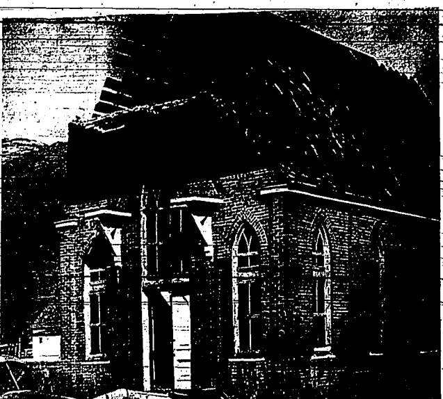
THE TRIPLE-THICKNESS of bricks in the gable ends of St. Francis Catholic Church in Bellevue are pushed out by Danny Ramsland and his helper as they worked to tear the building down. It has not been used since 1835. Ramsland said he and Harry Reese, both bricklayers, had purchased the building for the used brick and lumber. (Times-News photo)
