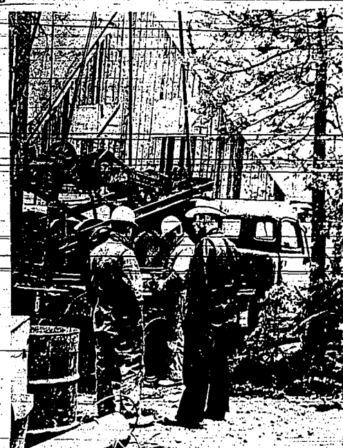
CONSULTING ON PROGRESS being made in digging a well at the 4-H camp being constructed up Quadrant Gulch, not far from Russian John ranger station, are from left, Darryl Smith, well driller, his helpers, Alan Devoe, and James Eakin. Blaine county agricultural agent in charge of operations, a good supply of water was reached at 60 feet, but the well will be driven deeper to obtain a 30-gallon per minute flow. (Times-News photo)
